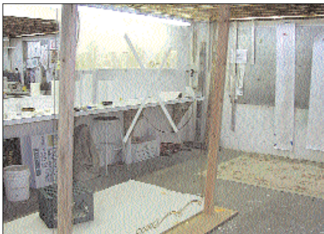
This photo shows the other panel of glass in the shop. The panel will receive the border treatment only. This will consist of 23-karat bright lines. The outside areas will be painted with lettering enamel just like the main panel.
