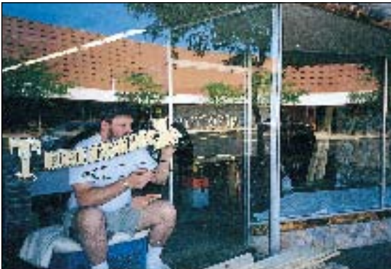
With the 23-karat bright lines already laid down, the centers of the letters were filled with a 16-karat matte center.
