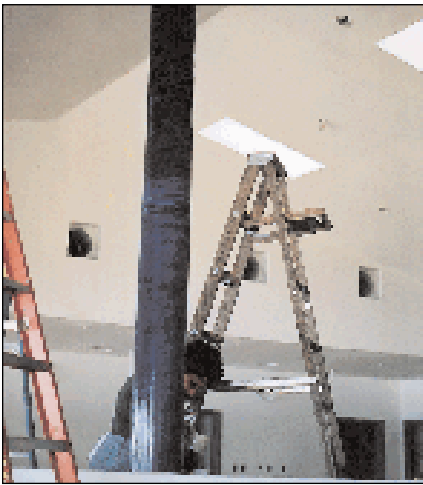
After being etched, primed and painted, we use large sponges to size the stovepipe.
