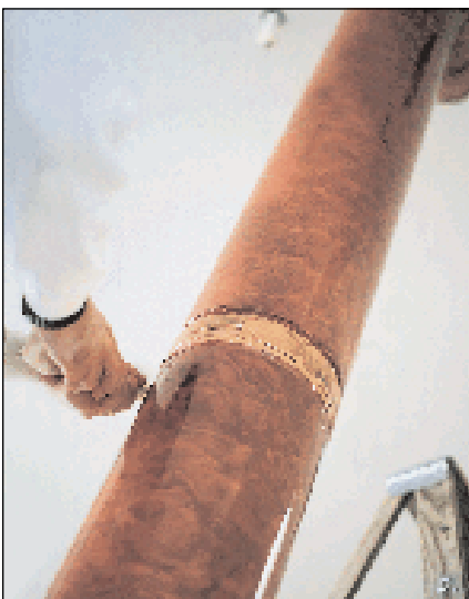
A toning glaze (color) is applied over the dry texture glaze. All color is removed from the coupling joints then clear coated, adding contrast and interest to the finished stovepipe.
