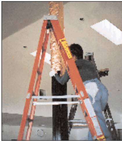
Working from 10' folding ladders, Robin and I work on opposing sides of the dividing wall. When working with copper leaf be sure to wear gloves — oil from your fingers will tarnish the copper.
