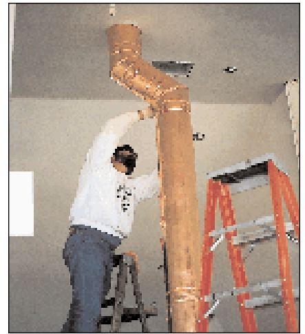
Using a foam brush, copper leaf is stomped into the cracks and joints.
