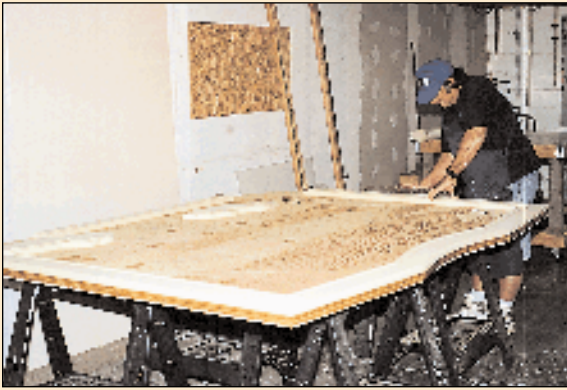
Marine-grade plywood was used as a sub-structure, making the over-sized measurements of 6' x 8' more user-friendly.
